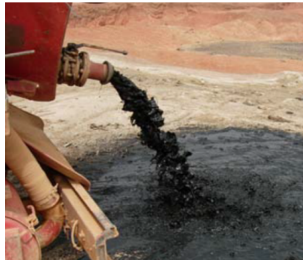
Figure 39: Septage being emptied at a FSTP
